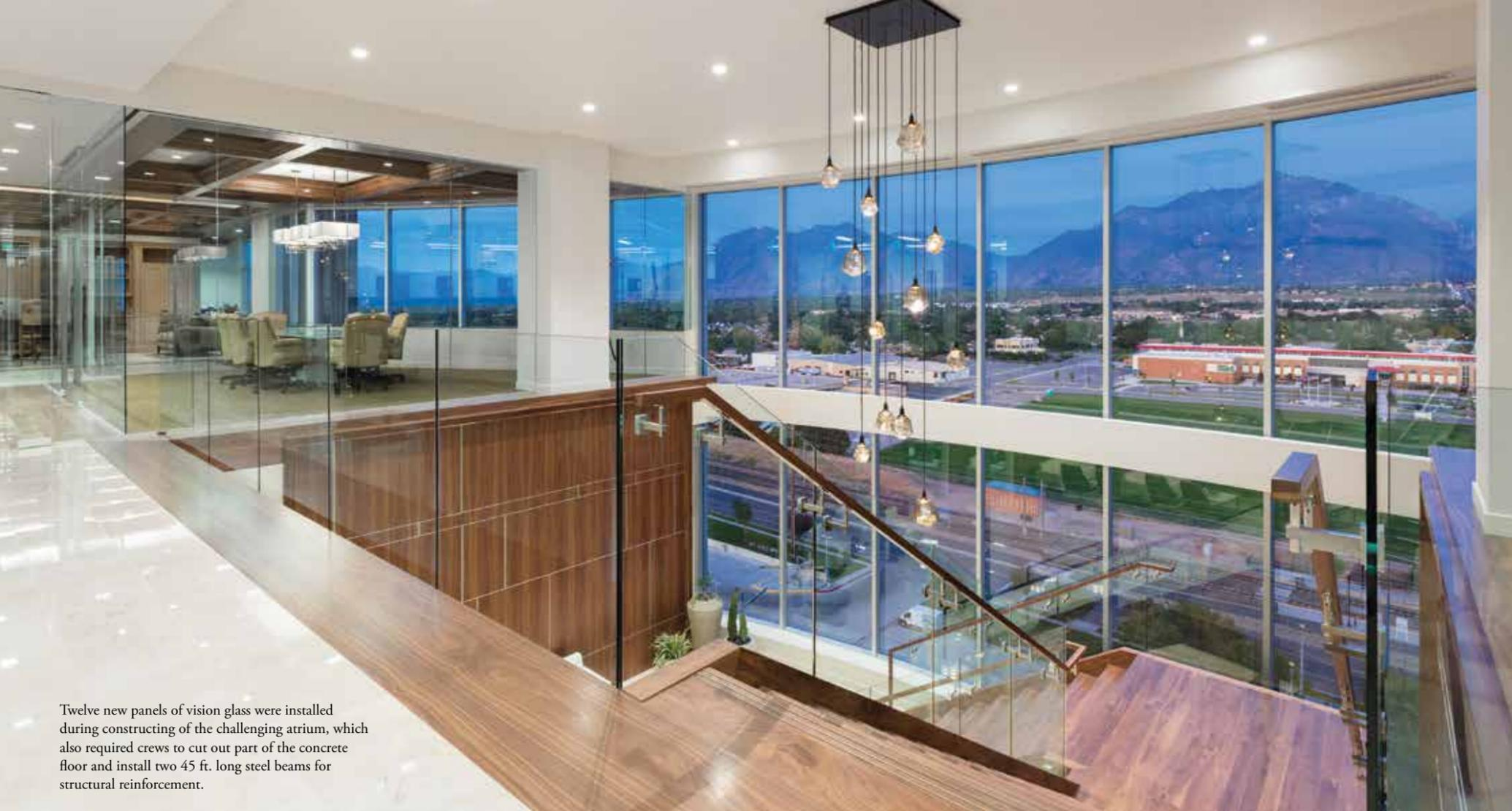
Twelve new panels of vision glass were installed during constructing of the challenging atrium, which also required crews to cut out part of the concrete floor and install two 45 ft. long steel beams for structural reinforcement.
